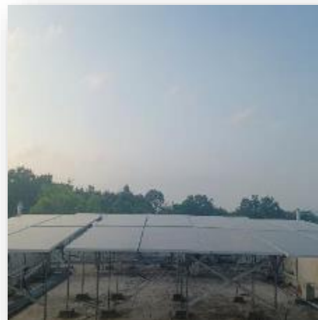
482 KWp Roof top Solar plats power Generating Power 1.5 to 2.35 MW/day
