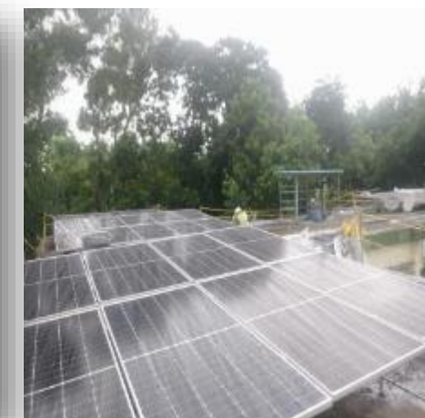
482 KWp Roof top Solar plats power Generating Power 1.5 to 2.35 MW/day
