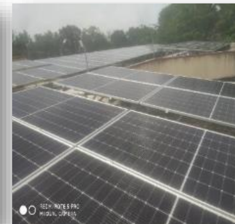
482 KWp Roof top Solar plats power Generating Power 1.5 to 2.35 MW/day
